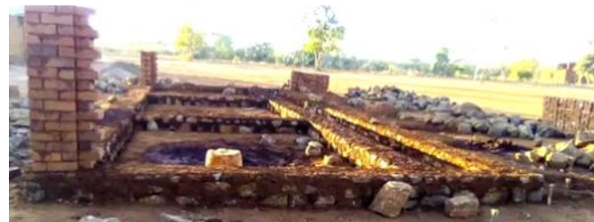
Building a foundation for a new housing unit at the Mananovy Bible School
