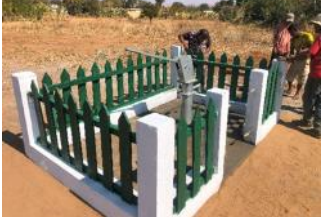
A new "Water Station" with a good hand pump built on top of a new well.
